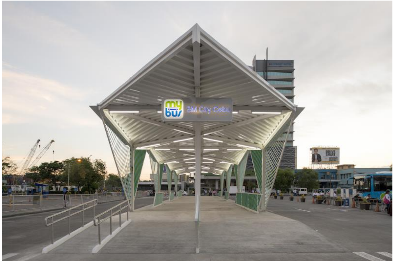
The roof of the bus stops is angled to deflect the heavy rain that Cebu experiences. The stormwater is directed to retention tanks. Image courtesy of CAZA
